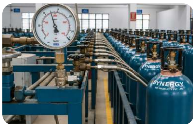
Argon (Ar) Welding & specialised processes
